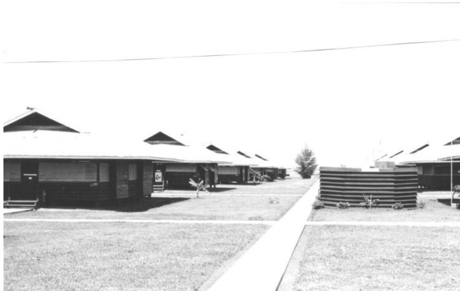
Photo Image 2 - Open air hootches with central latrine
