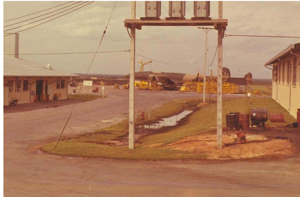
Photo Image 3 - Toxic Chemical drums (barrels) near EMS Shops
