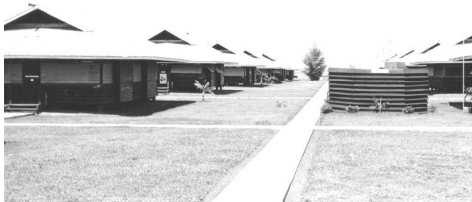
Photo Image 2 - “Hootch” type living quarters near perimeter
